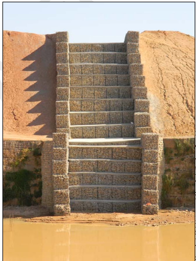
View of the stepped gabion structure
