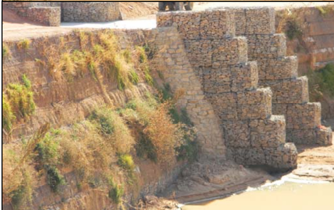
Views of the smaller stepped gabion structure
