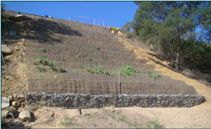
PHOTO 3 - Front View of the completed structure
