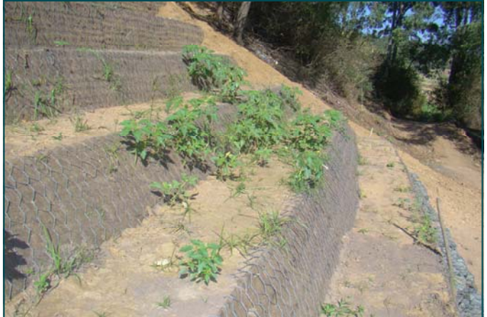
PHOTO 4 - Vegetation establishing naturally
