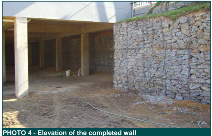
PHOTO 4 - Elevation of the completed wall
