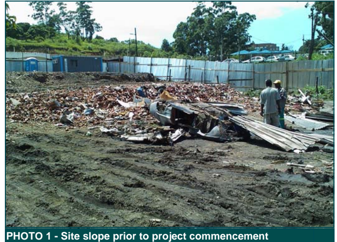
PHOTO 1 - Site slope prior to project commencement
