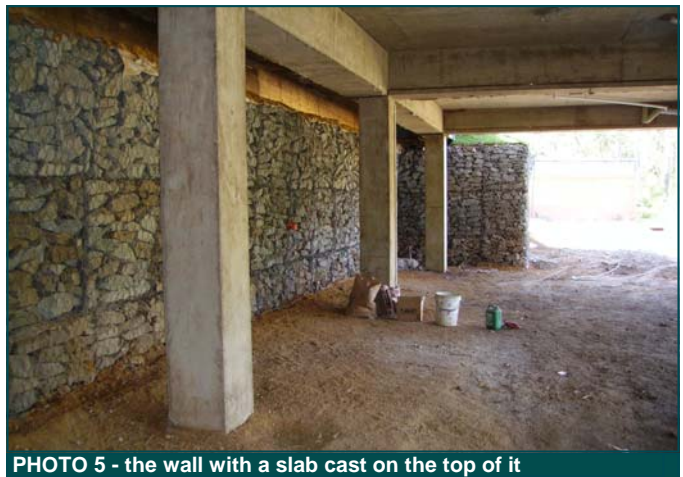
PHOTO 5 - the wall with a slab cast on the top of it
