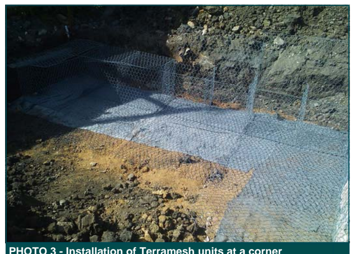
PHOTO 3 - Installation of Terramesh units at a corner
