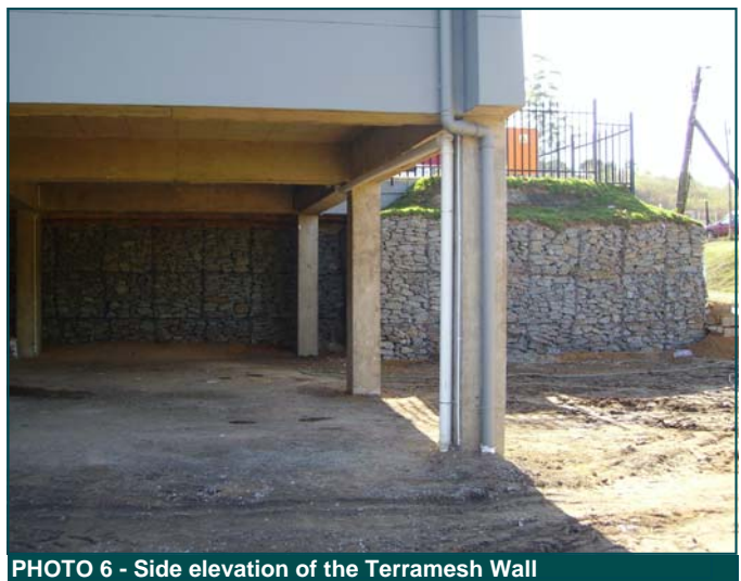
PHOTO 6 - Side elevation of the Terramesh Wall
