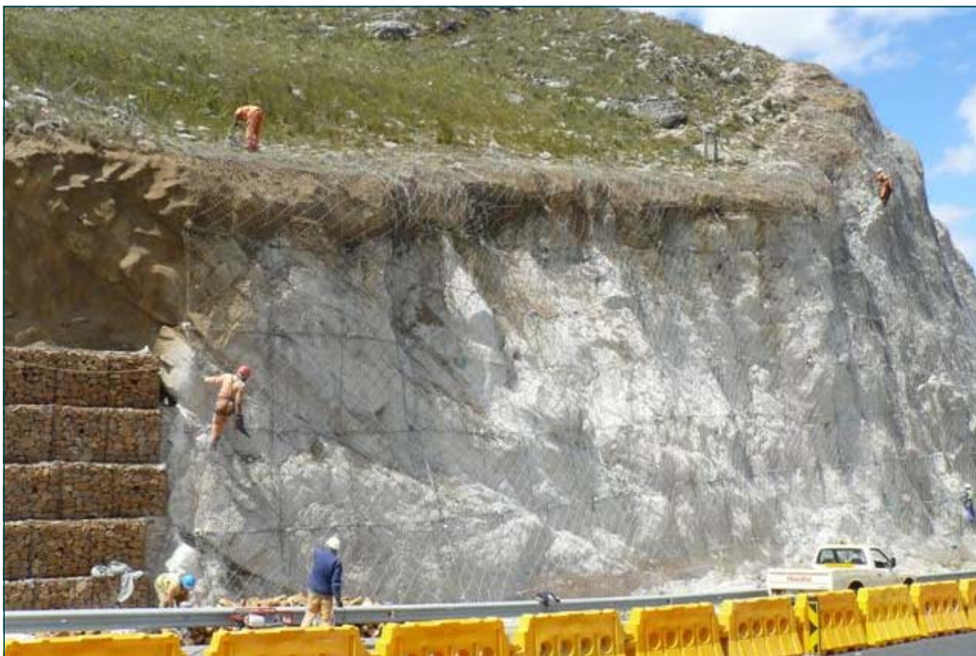
Combination of HEA / Drapery mesh anchored to the face
