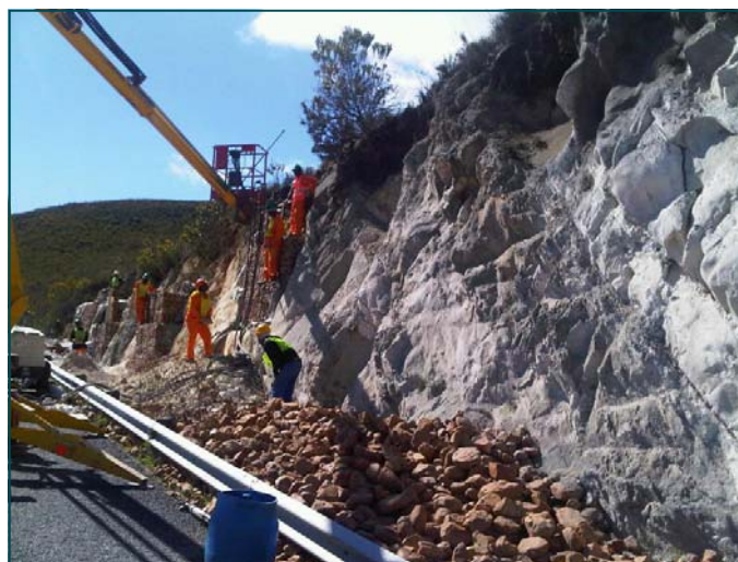
Gabions walls completing the lower section
