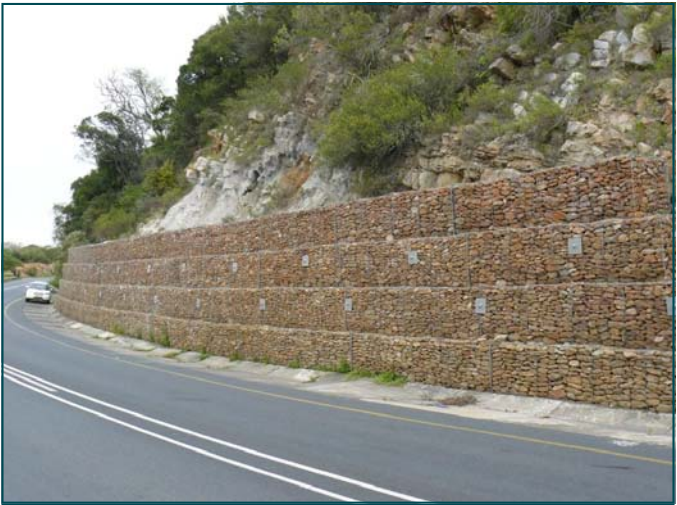
Solution provides both slope stabilisation and rock debris trap
