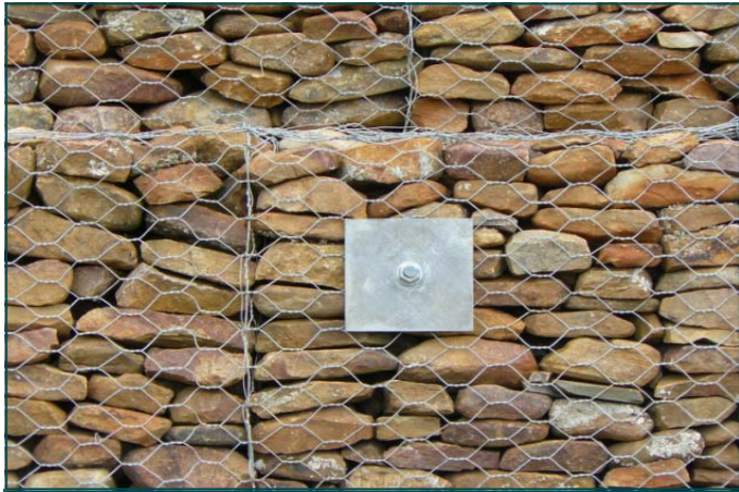
Rockbolt anchor support fixing gabions into the cutface rockmass
