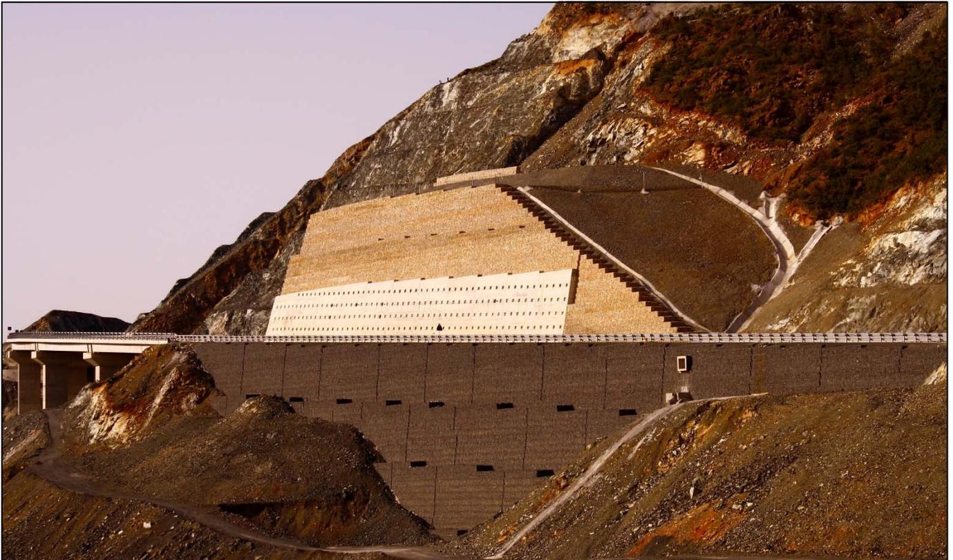
Completed reinforced soil structure with slope stabilisation measures above highway
