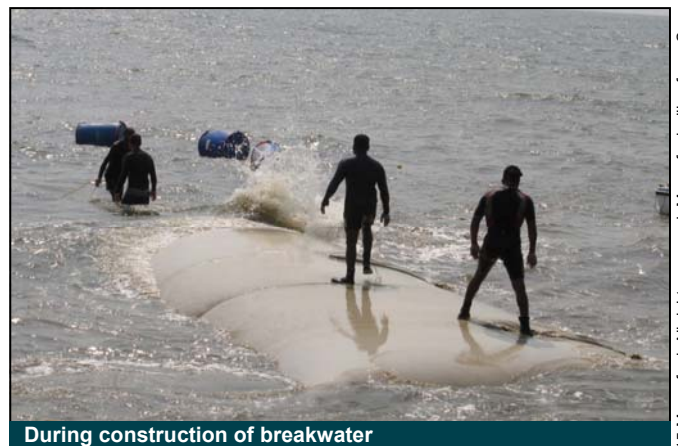
During construction of breakwater
