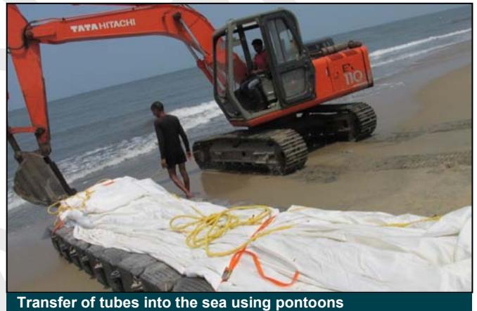
Transfer of tubes into the sea using pontoons
