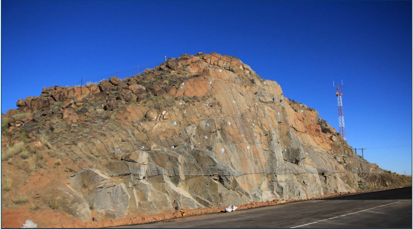
Complete face with anchors & SteelGrid® HR 50
