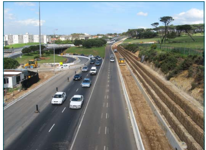
PHOTO 1 - Showing progress of construction
