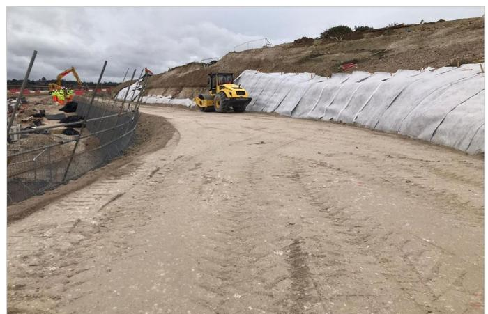
Cement improved chalk as structural backfill
