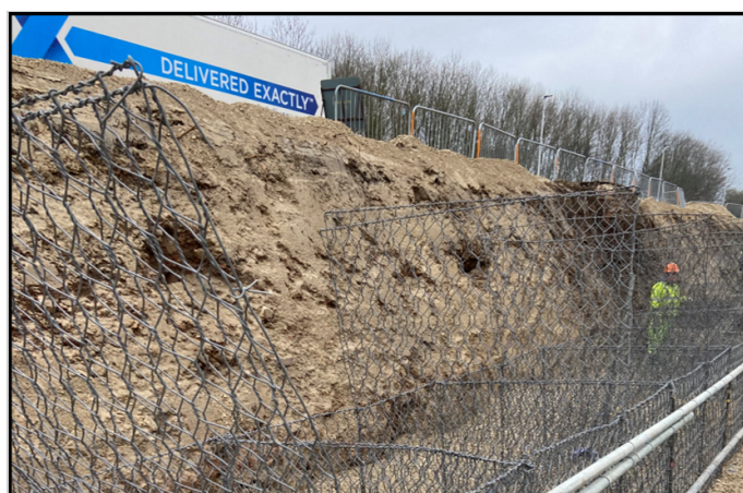
Gabion units laid out ready for filling - note highway above
