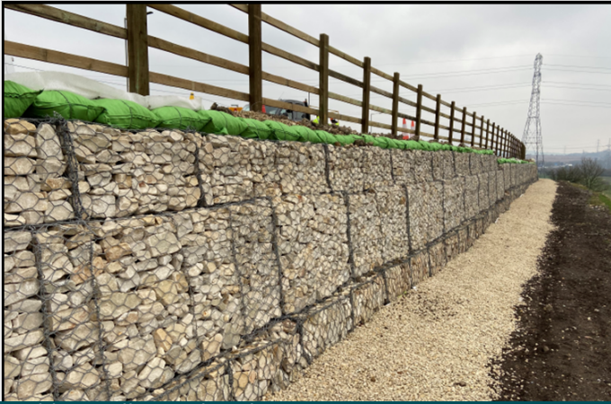
Gabion wall completed
