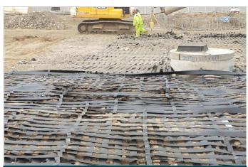
Layers of ParaLink® can be installed perpendicular to ncrease protection
