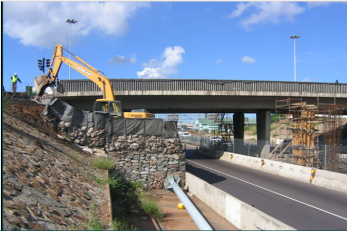
Temporary Gabion Wall
