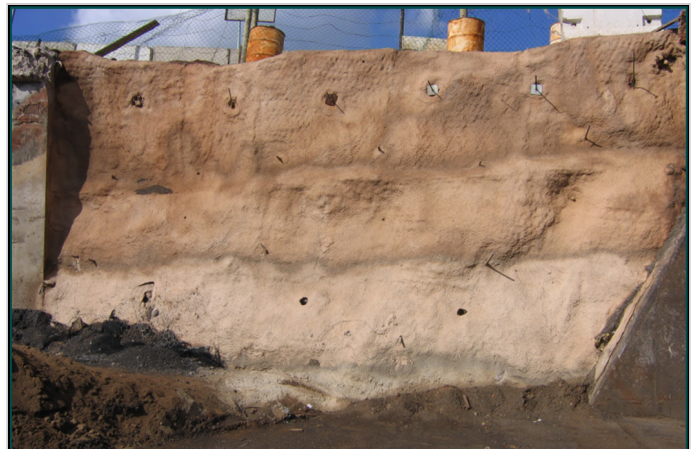
Finished soil-nailed and shotcreted face
