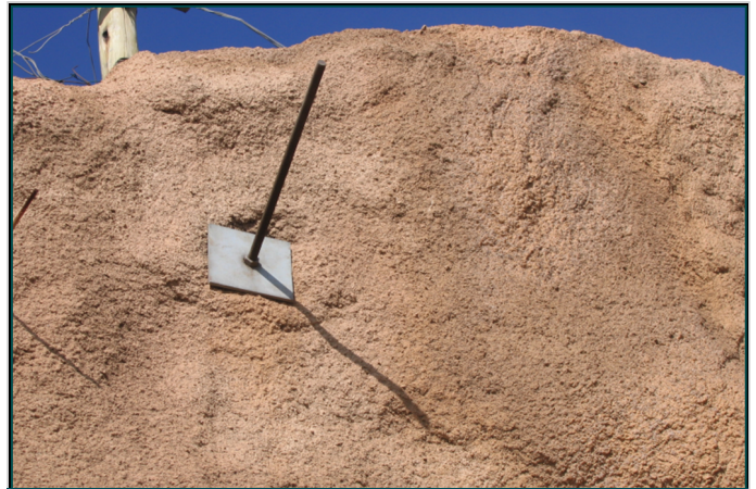
Installed Soil Nail
