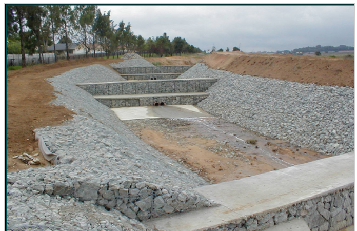
Gabion weirs to dissipate energy and protect the bed canal
