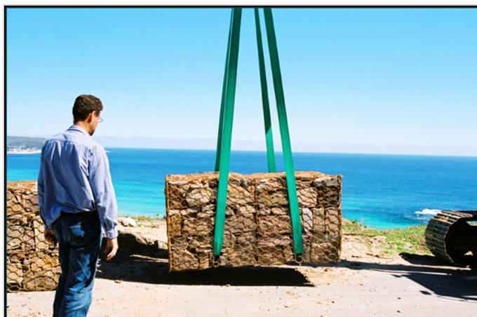
Prefilled units, with PVC pipes, lifted off the ground
