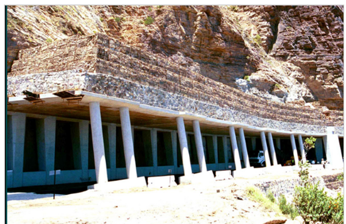
Canopy with gabion impact barrier above
