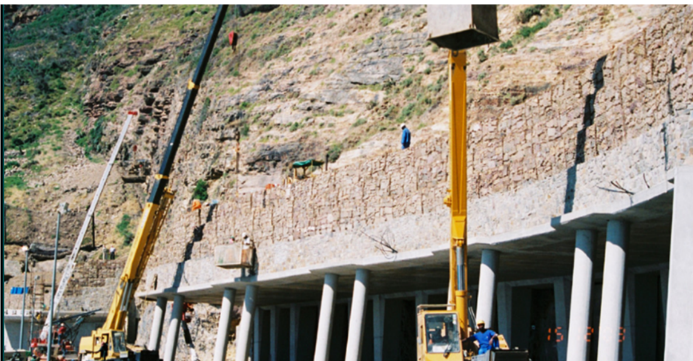
Backfill soil being lifted to fill behind gabions
