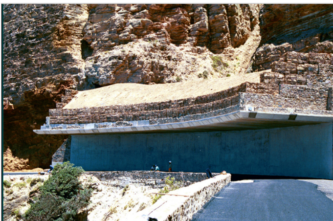
Cantilever structure with gabion impact barrier
