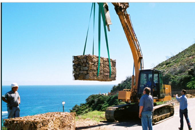
Lifting the prefilled unit
