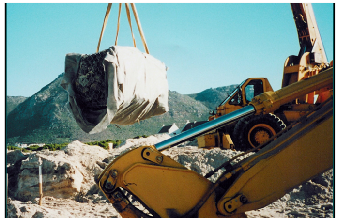
Lifting the prefilled units
