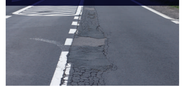
Fatigue cracking
