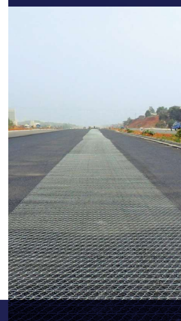
Road Mesh® - Structural reinforcement of asphalt
