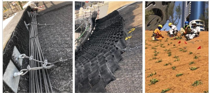
Macmat HS & Concrete Anchor Installation
