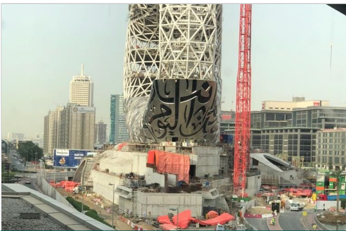
During construction: embedded building before covering with green cladding
