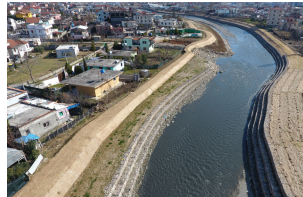
Channelling works containing river in urban area
