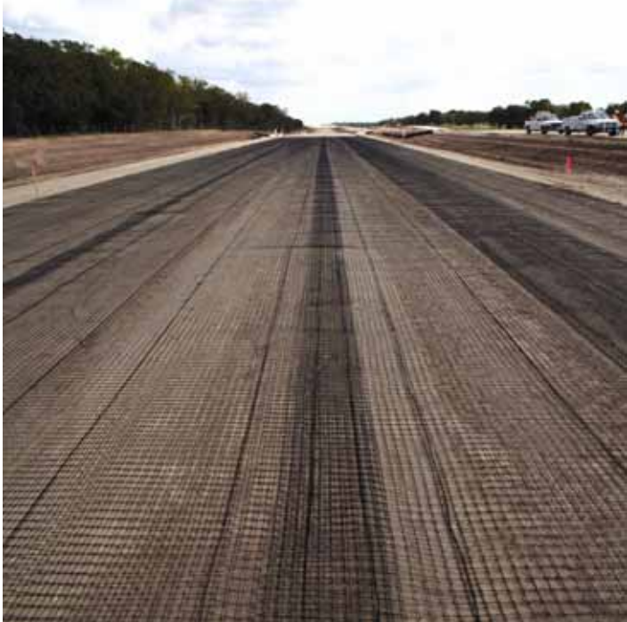
Recent View of the Structure
