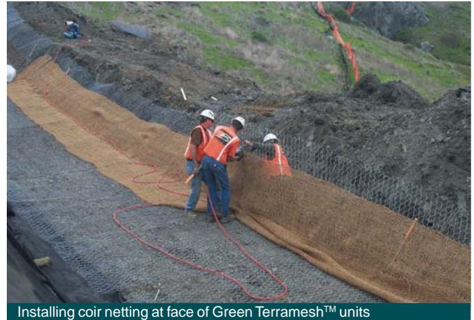
Installing coir netting at face of Green Terramesh™ units
