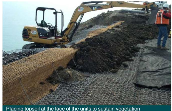
Placing topsoil at the face of the units to sustain vegetation
