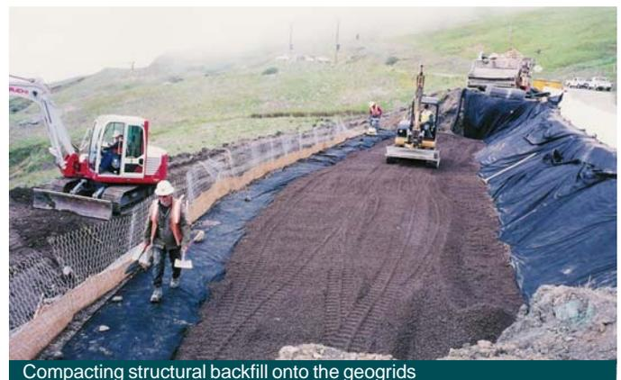
Compacting structural backfill onto the geogrids
