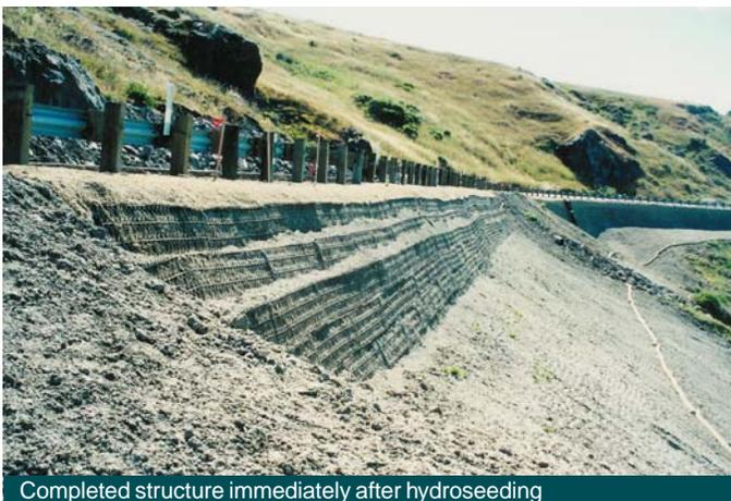
Completed structure immediately after hydroseeding
