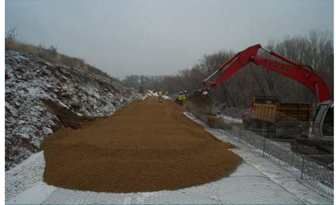
Placement of structural backfill onto geogrid reinforcement
