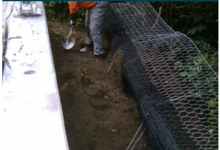
Green Terramesh® being filled with soil.
