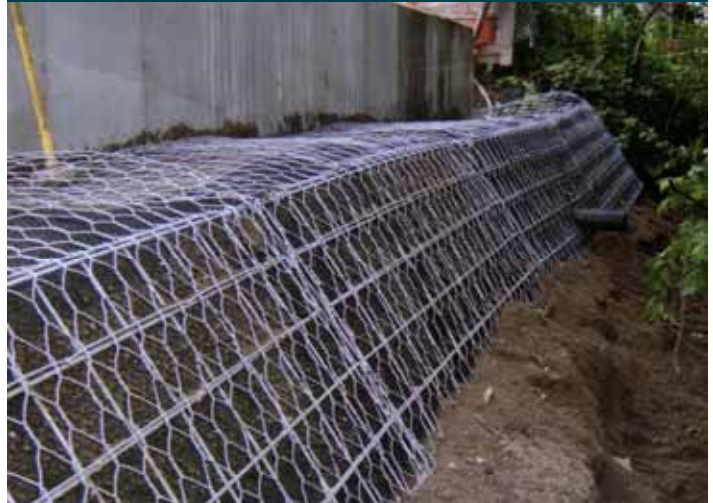
Completed Green Terramesh® waiting for hydroseeding.
