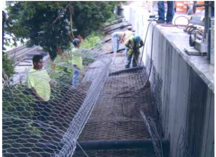
Green Terramesh® being installed at the base of the exposed footing.
