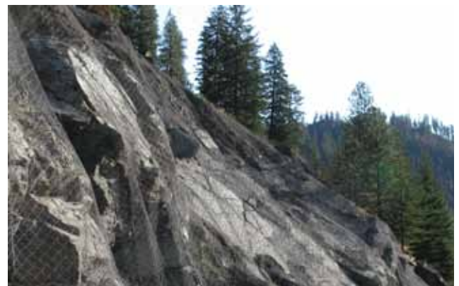
Maccaferri HEA Panels Installed
