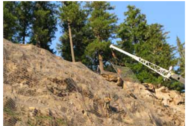
Installation of Maccaferri HEA Panels
