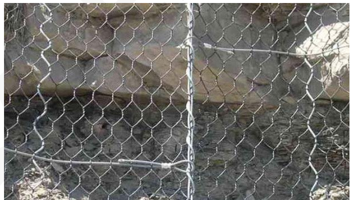
Lacing cable at every mesh opening
