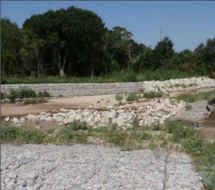
Gabion wall protecting the bank and Gabion Mattresses protecting the channel bed
