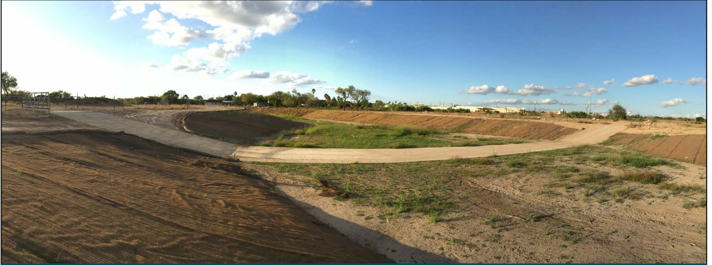
Completed site following installation of BioMac Turf Reinforcement Mat
