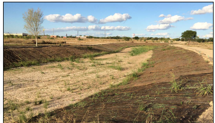
Images following installation with vegetation growth
