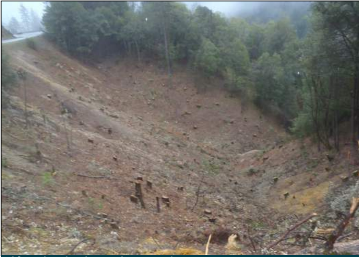
After site clearing and preparation
