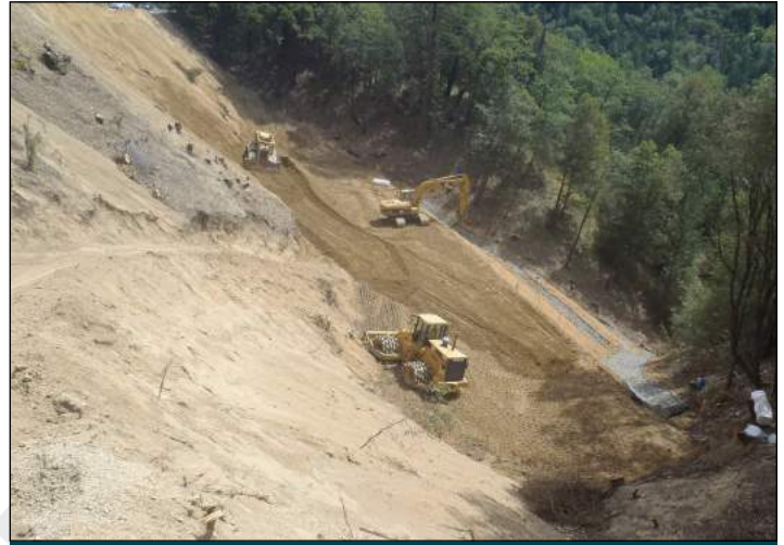
Installation of the benches
