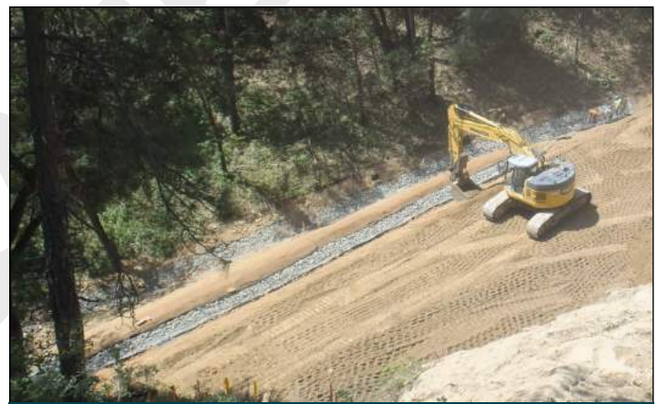
Installation of the Gabion Benches
