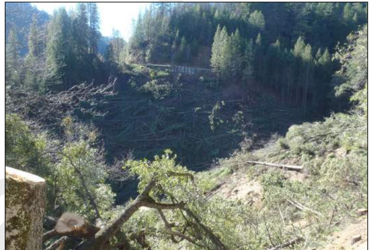
Site Prior to Work
