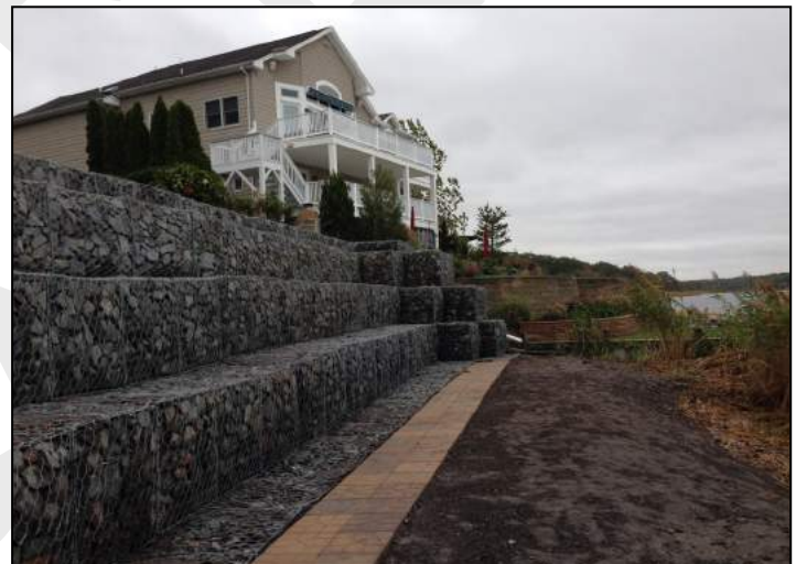
Post installation- completed wall
