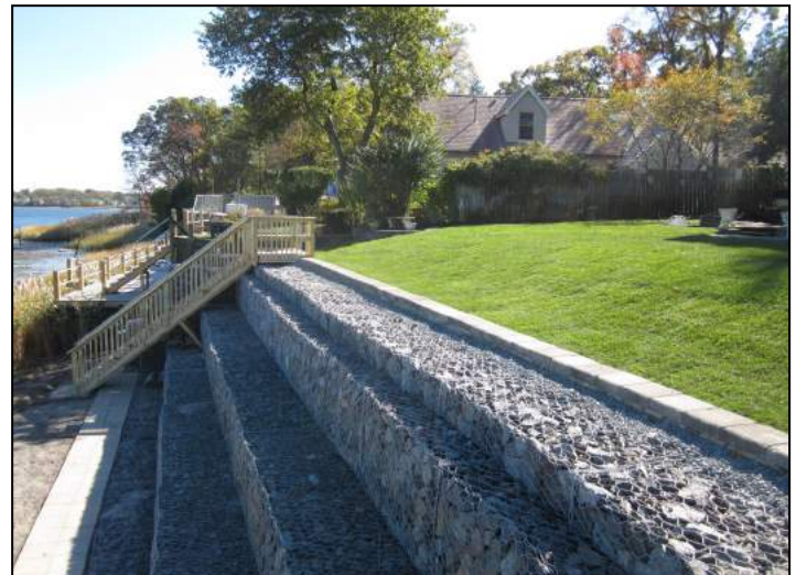
View of completed project approximately 1 year after installation.
