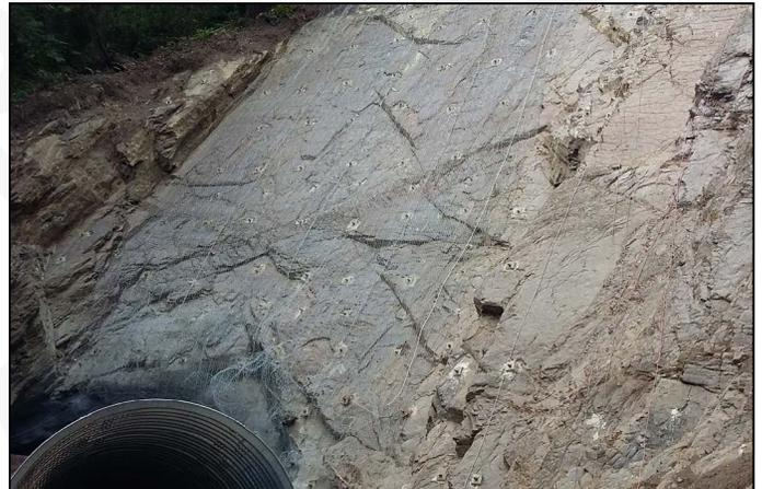
When a second and third rockfall event occurred in June, more material was immediately shipped to the construction site and had to be hung the day it arrived. Maccaferri assisted the freight company to bring the material to the remote jobsite.
