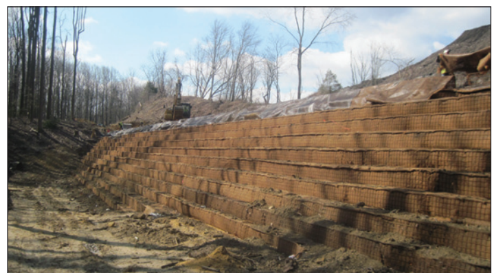
Front view of the MSE wall under construction
