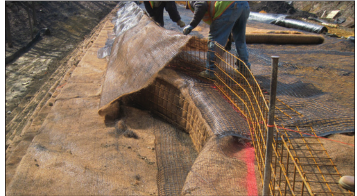
Attaching BioMac® and MacGrid® WG to the fascia
