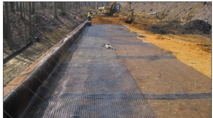
Placing backfill over MacGrid® WG
