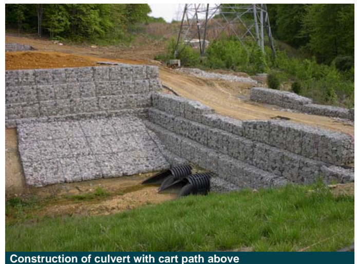
Construction of culvert with cart path above
