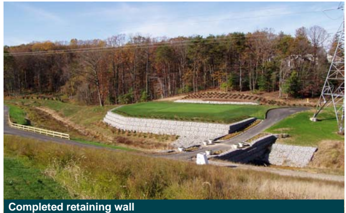
Completed retaining wall
