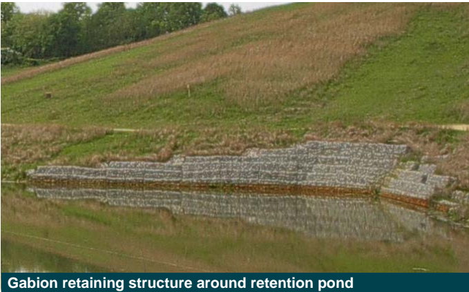
Gabion retaining structure around retention pond
