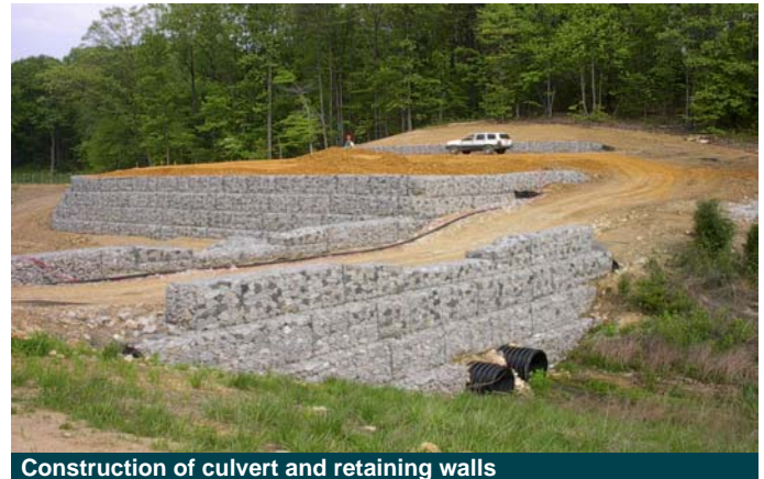
Construction of culvert and retaining walls
