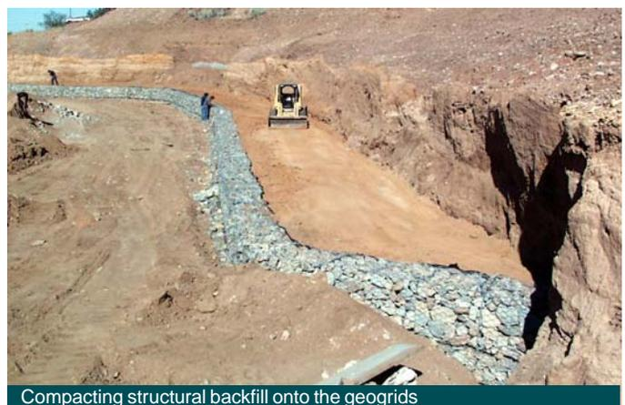
Compacting structural backfill onto the geogrids
