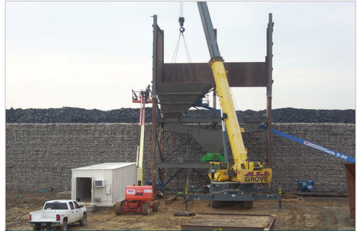
Installation of Dual Hoppers
