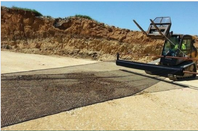
MacGrid® WG15 installation - rolling out the grid
