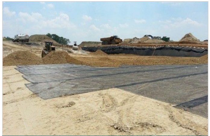
MacGrid® WG15 installation - backfilling
