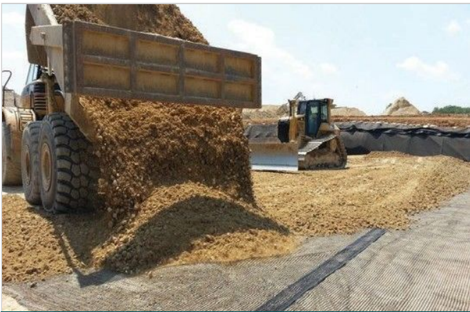
MacGrid® WG15 installation - backfilling
