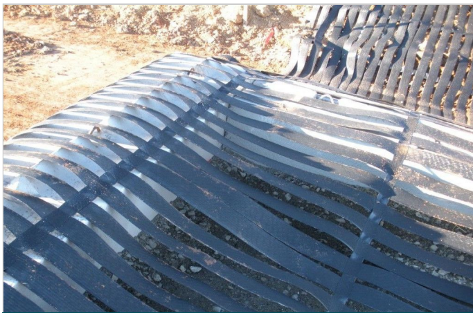
Wrapping the Blocks - 15' minimum
