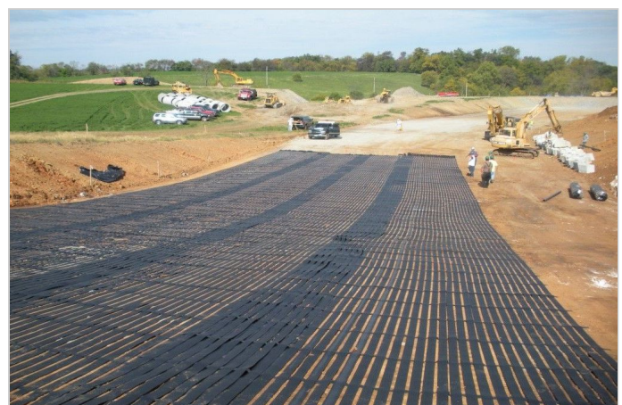
During construction - First layer installation
