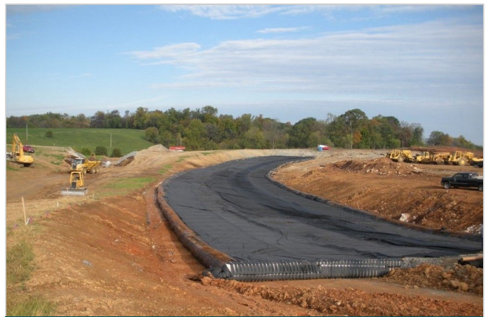
ParaLink Completely Installed
