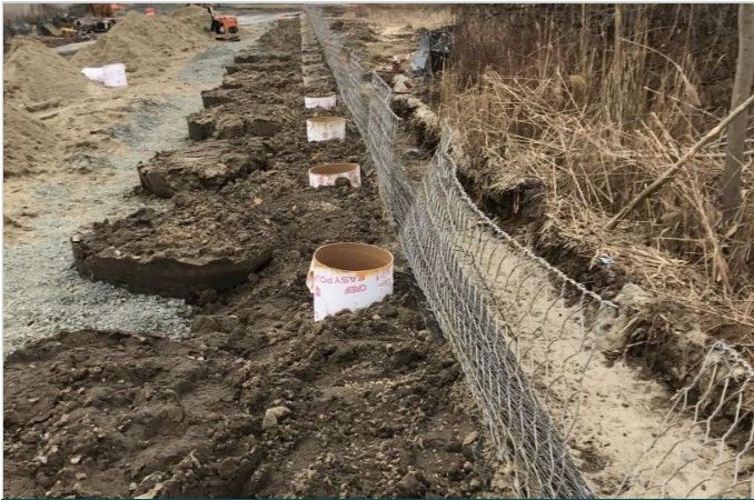
Sonotubes embedded in the wall for guardrail installation
