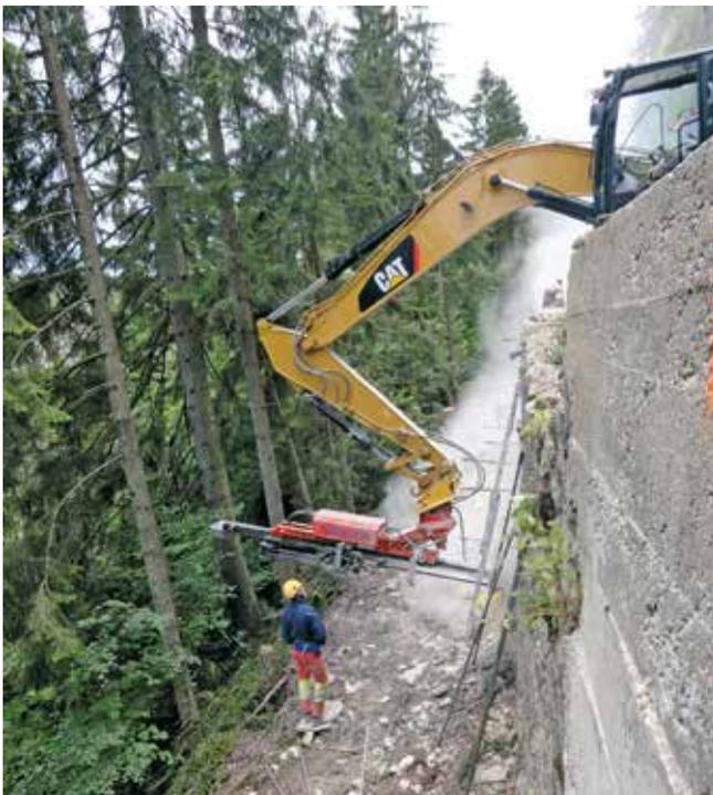
Anchor holes being drilled in a construction project
