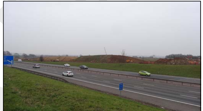
Site won-fill material stockpiled - view of the site in April 2016
