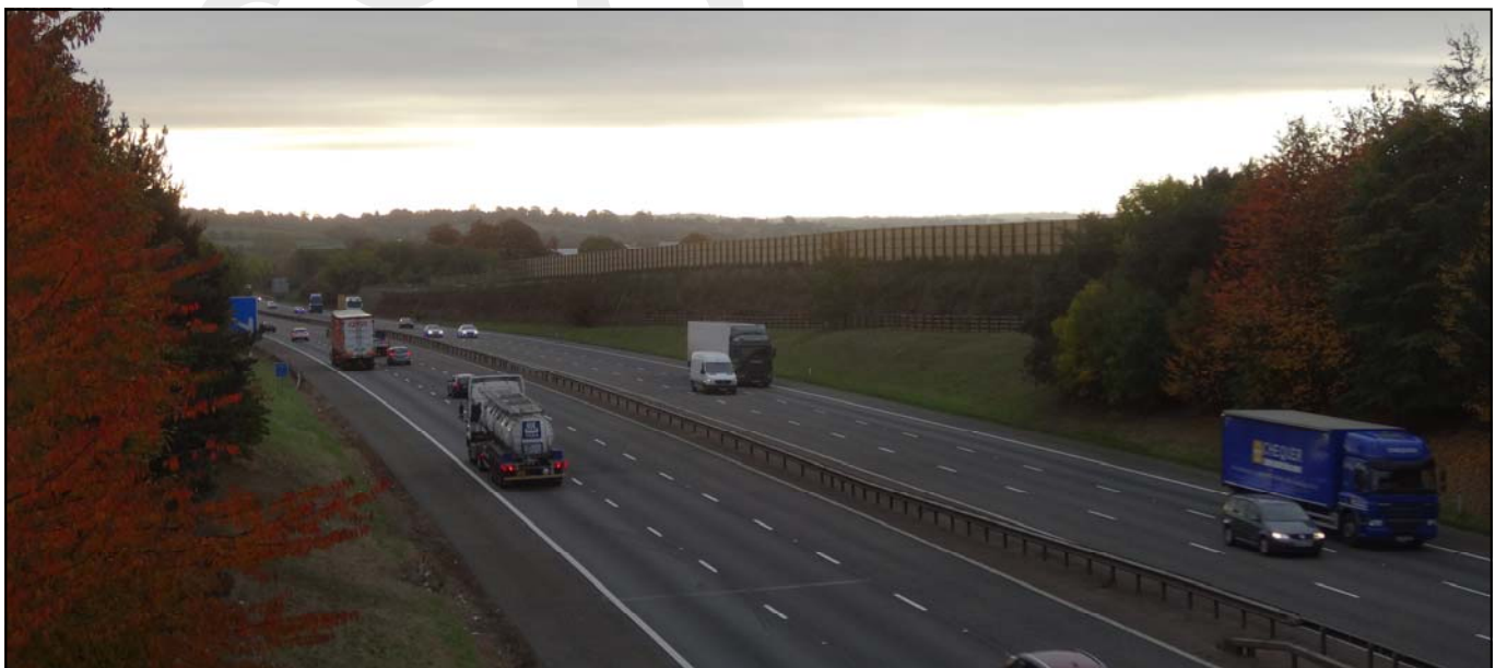
View of the acoustic barrier facing the M40 - October 2016
