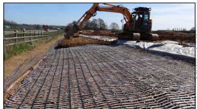
Placing of the poor marginal backfill over the Paradrain
