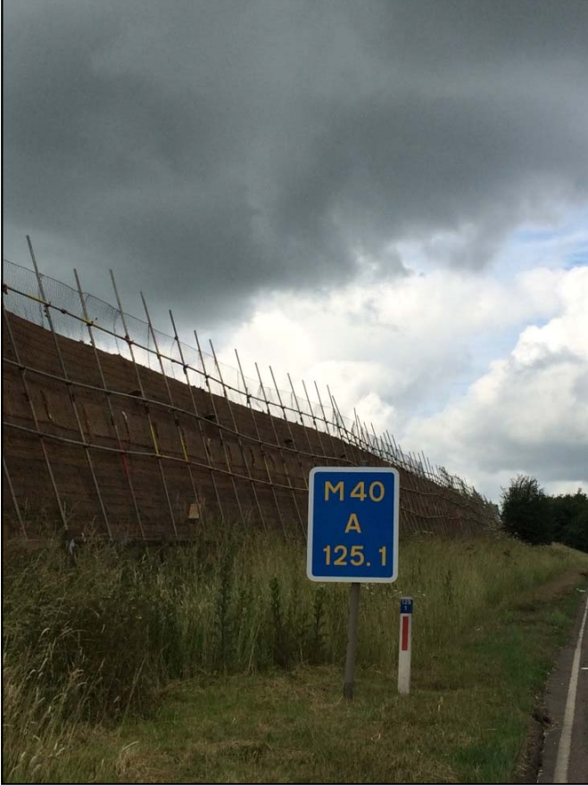
View of the 70 degree Green Terramesh with edge protection
