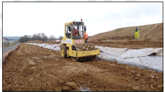
Cohesive fill material compacted with sheep foot roller
