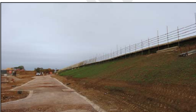
Rear of the bund with 1:3 slope allowing landscaping
