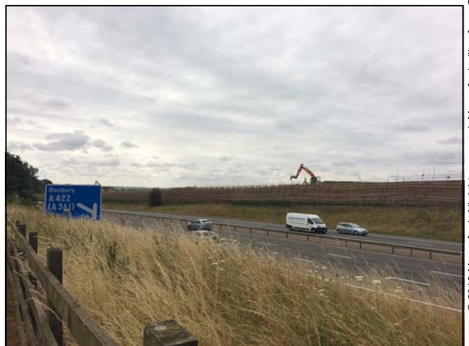
View of the structure in July 2016
