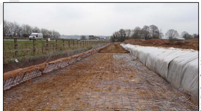
Green Terramesh, Paradrain and Macdrain - initial phases
