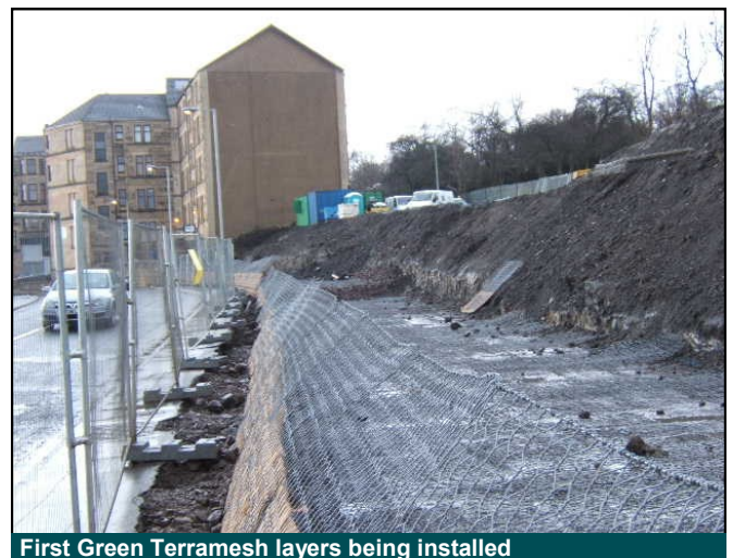
First Green Terramesh layers being installed
