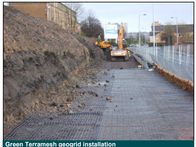
Green Terramesh geogrid installation
