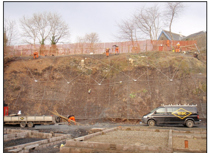
Completed works including external rope network
