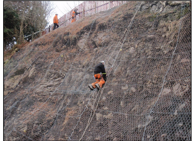
Installation in progress
