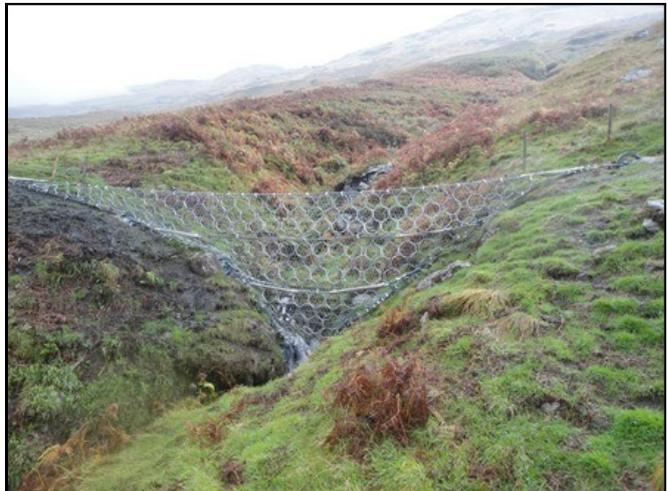
View of fence B in installed position—note lack of posts
