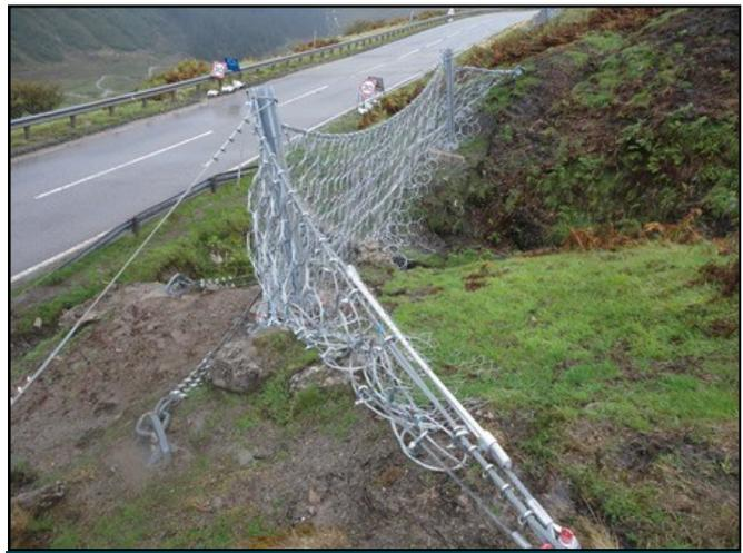
View of fence C following installation showing curved layout
