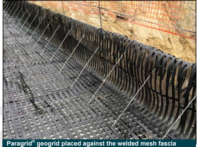
Paragrid® geogrid placed against the welded mesh fascia
