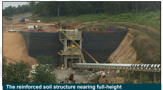
The reinforced soil structure nearing full-height
