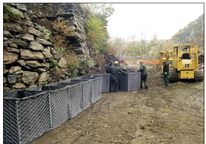
Installing additional lengths of FlexMac® DT
