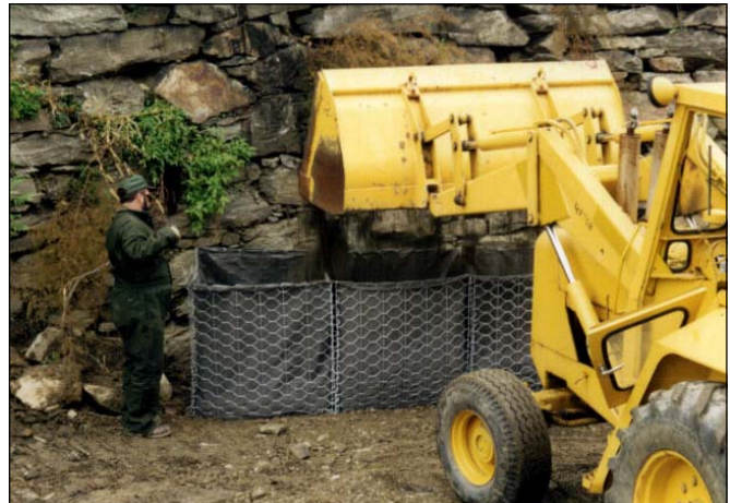
Filling additional lengths of FlexMac ® DT
