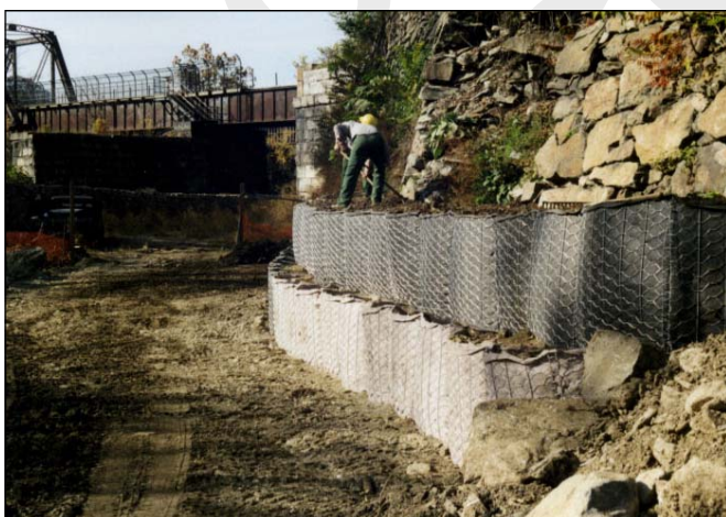
The second of three layers nearing completion
