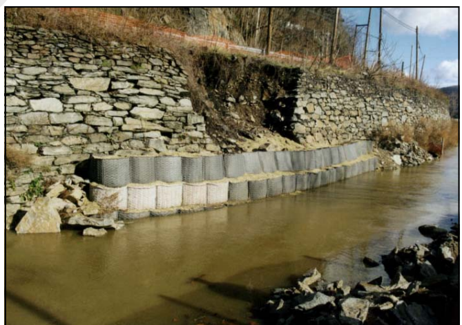
Canal filled after completion; First 1m course is submerged
