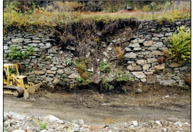
Site preparation for the temporary wall
