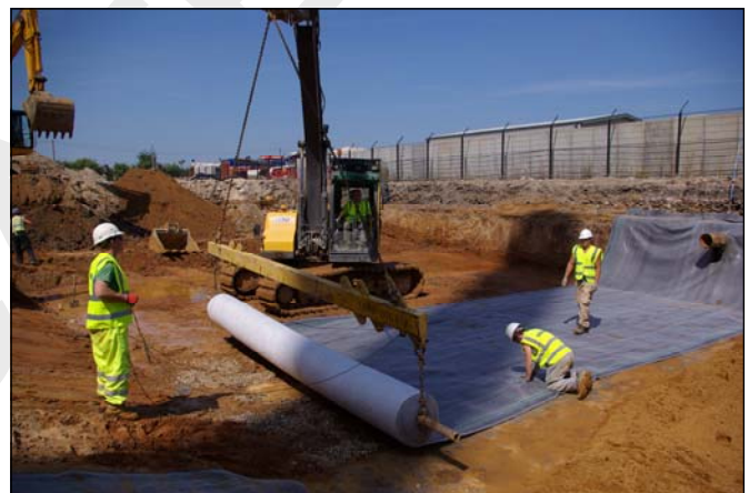
MacLine® during installation
