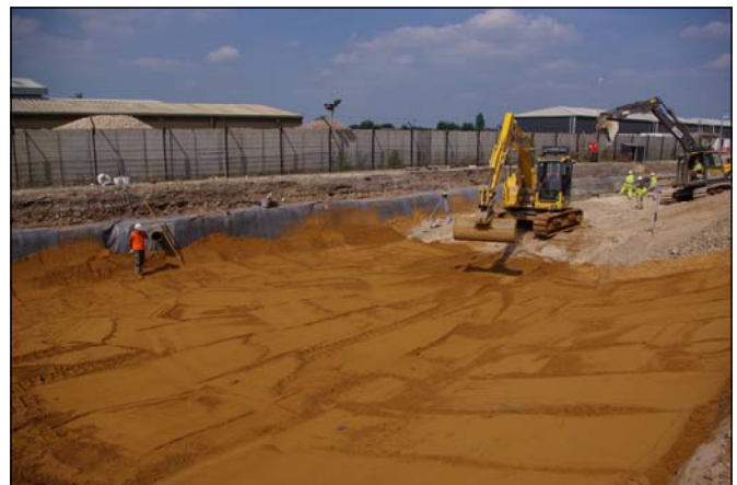
MacLine® and Gabion installation
