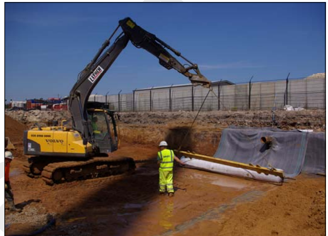
MacLine® during installation
