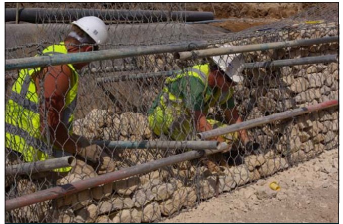
Installation of double twist gabions
