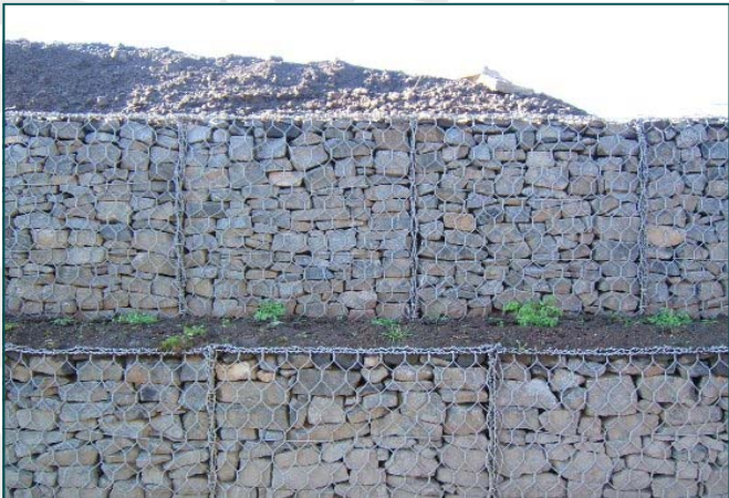
Vegetating gabion terraces
