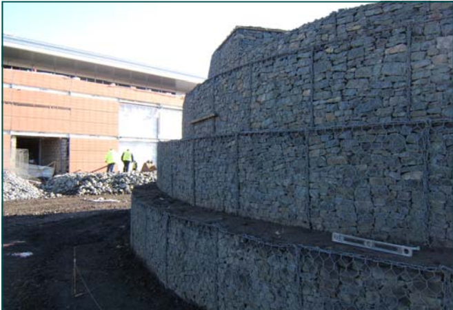
Curved gabion retaining wall
