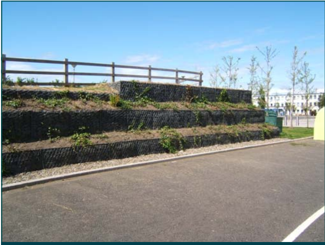
Completed entrance wall
