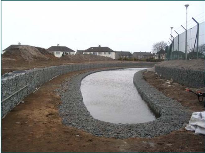
SUDS Pond gabion walls completed
