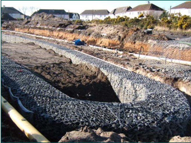
SUDS Pond gabion walls under construction
