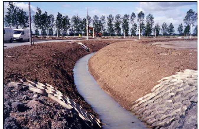
Topsoil placed into cells
