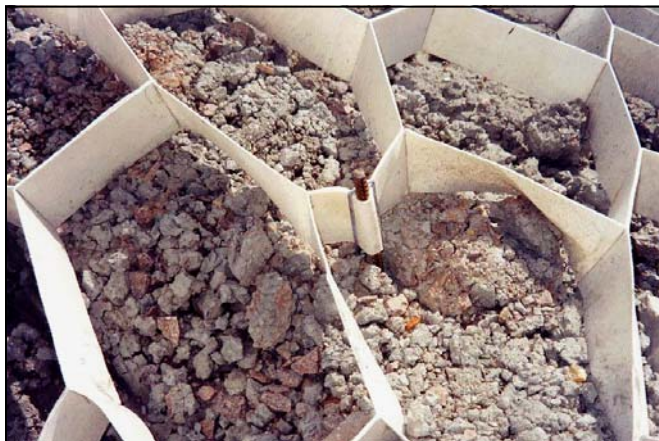
Macweb and fixing pin detail
