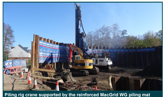
Piling rig crane supported by the reinforced MacGrid WG piling mat
