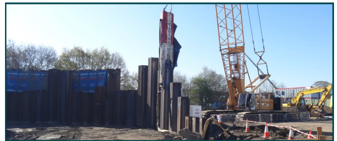
The Liebherr crane supported by the reinforced MacGrid WG piling mat
