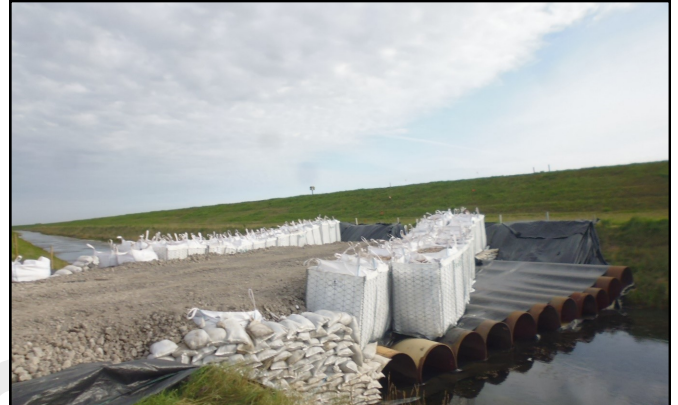
Initial phases of the works
