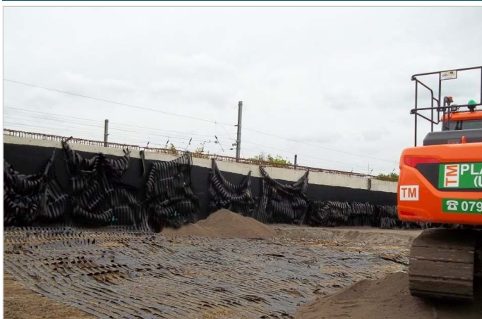
Paralink being laid flat and wrapped back as per design
